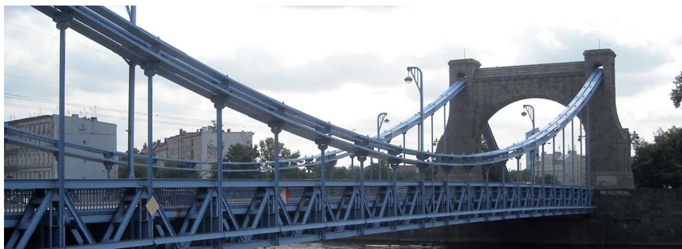
This is one of the 106 bridges in Wrocław. It is unique in that it is built without the use of a single screw. The river is the Oder.
